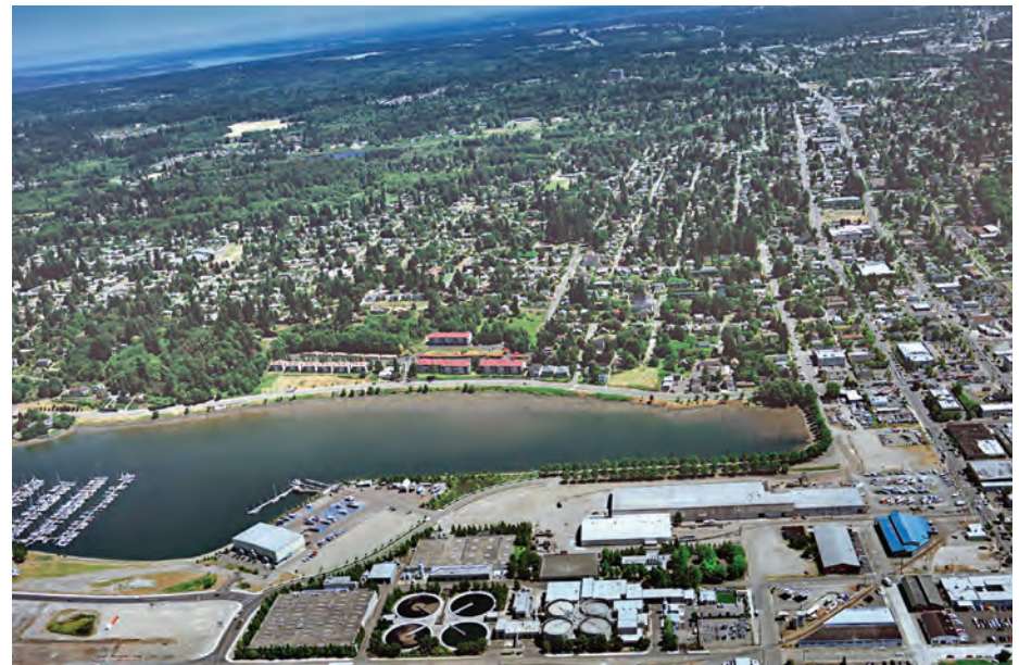
Photo courtesy of Washington State Department of Transportation.
