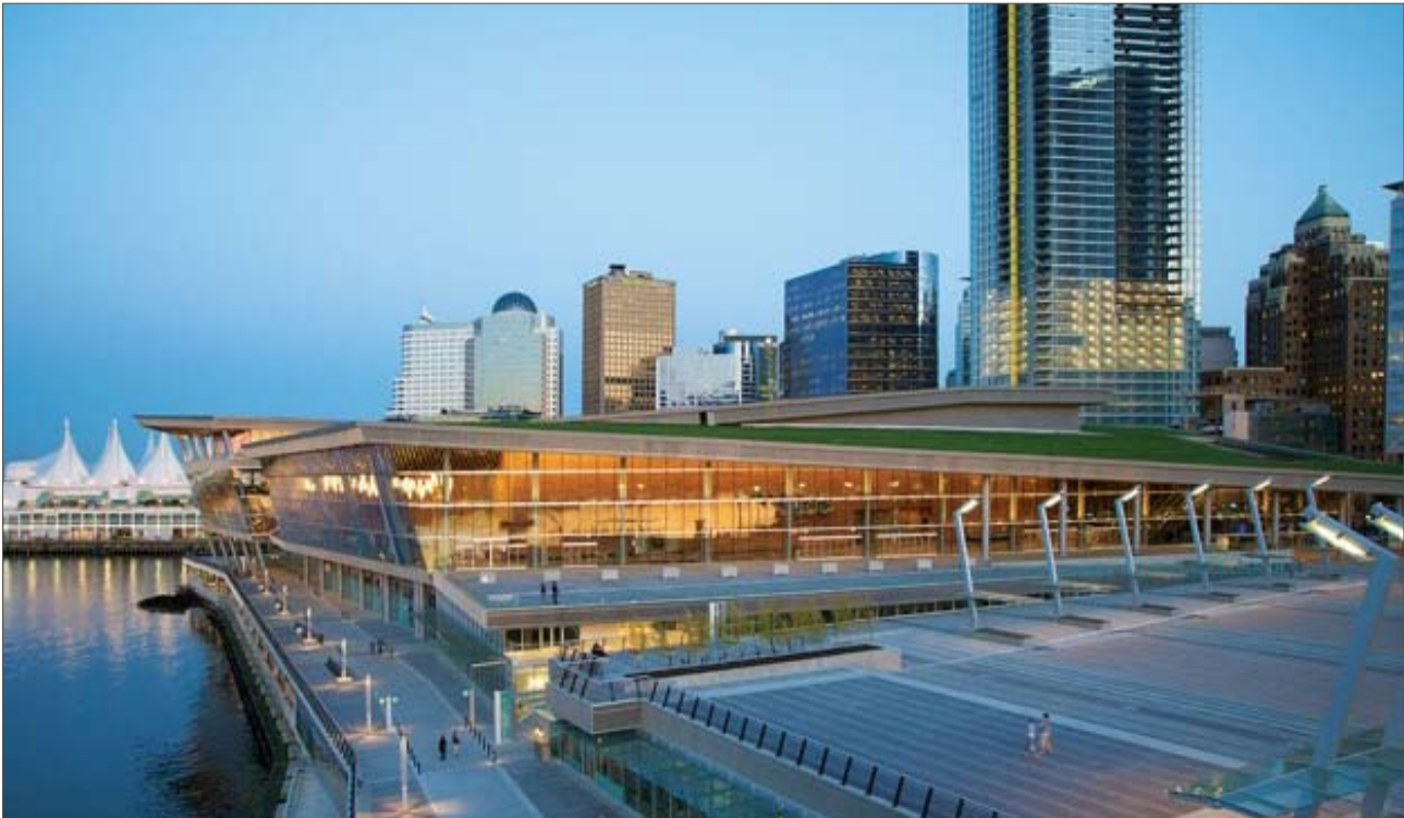
The Convention Center in downtown Vancouver, British Columbia, houses a membrane bioreactor designed to treat 20,000 gallons of wastewater generated by the facility each day. All of the building's treated wastewater is recycled onsite for flush fixtures and to irrigate a six-acre green roof.
