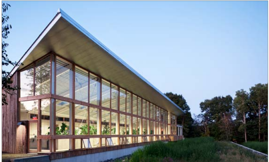
The Omega Center for Sustainable Living in Rhinebeck, New York, is one of the first projects certified under the Living Building Challenge. The project is a wastewater filtration facility designed to reuse treated water for irrigation and serve as a teaching tool for campus educational programs. Image: Farshid Assassi courtesy of BNIM Architects
