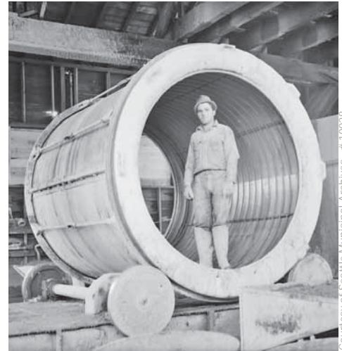
Six foot diameter sewer pipe, 1935.
