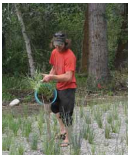
Constructed wetland in Sun Valley achieves high levels of water quality before infiltrating the processed wastewater at a location close to its source.
